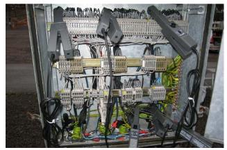
Figure 3 Control cabinet with current clamps
